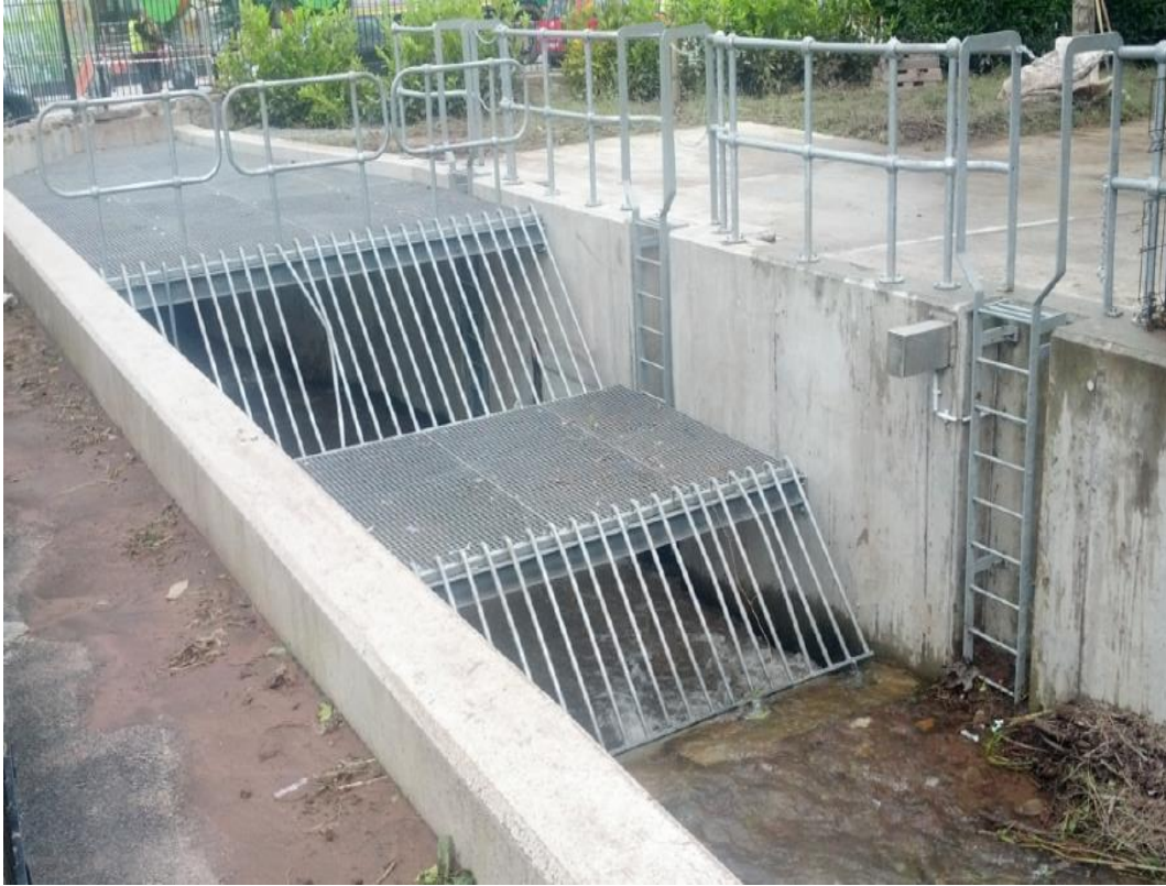
Figure 2.4: Church Road culvert trash screen – normal conditions. Source: OPW
