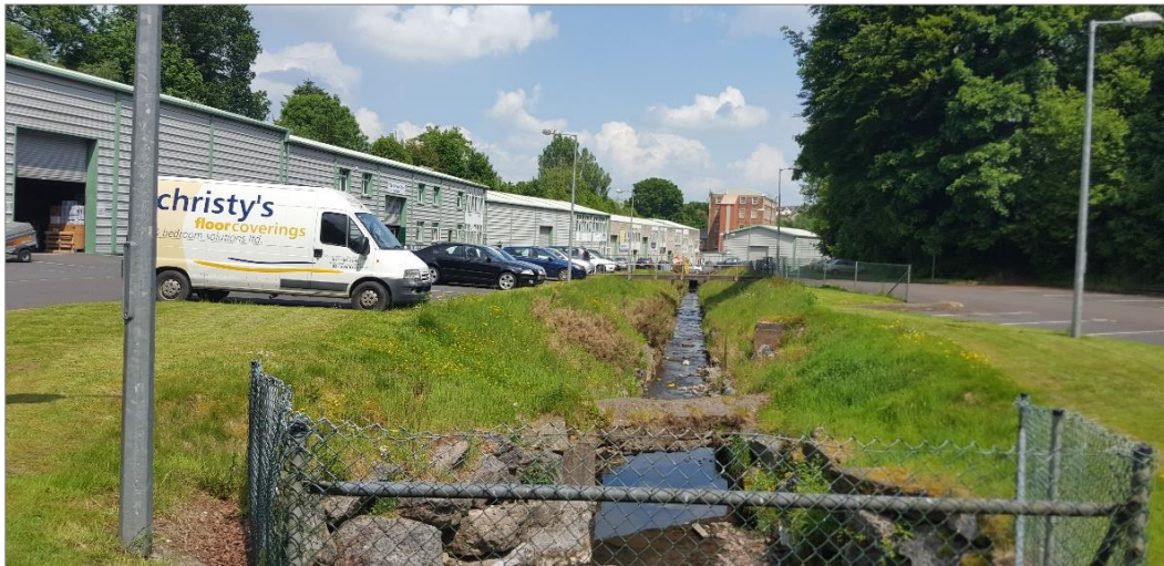
Figure 7.3: View north-east through Donnybrook Commercial Centre, with existing open channel (Grange Stream) running down the central car park area of the complex, the mixed use units visible on the left, and the protected red-brick mill structure visible off centre right background.
