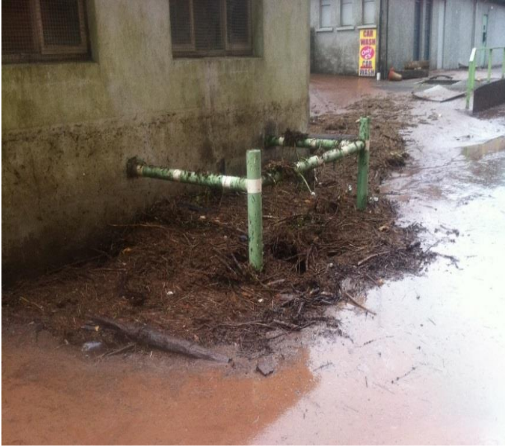
Figure 2.12: Post 2012 flood event at Donnybrook Commercial Centre showing debris at manhole. Source: Donnybrook Commercial Centre
