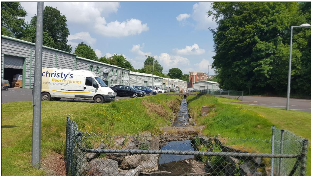
Figure 3.10: View north-east through Donnybrook Commercial Centre and Grange Stream.
