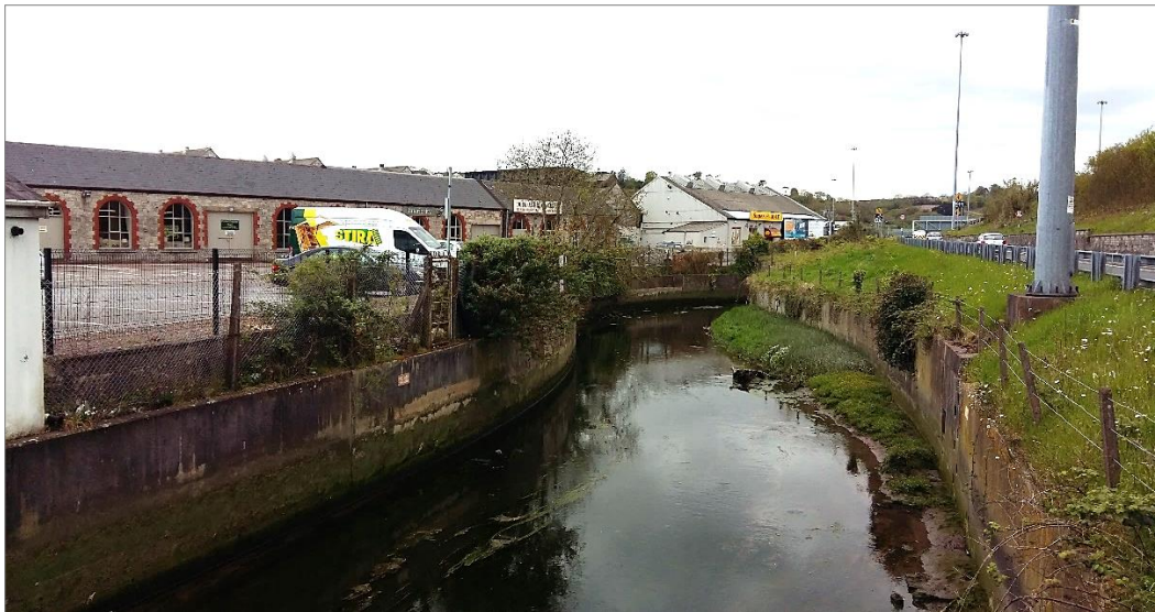
Figure 7.1: View of proposal site from R851, along open culvert on Tramore River, adjacent to St Patrick's Mills on the left and a slip road to the N40 on the right.
