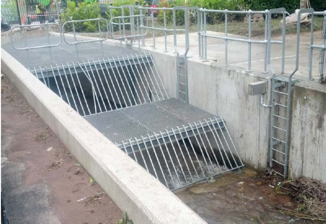
Figure 8.4: Church Road culvert trash screen – normal conditions. Source: OPW
