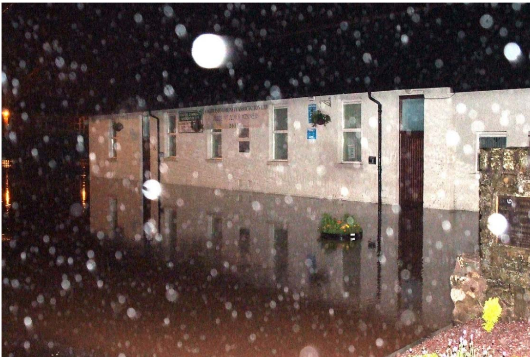
Figure 8.16: Post 2012 flood event in Togher Area – outside Togher Community Centre. Source: Cork County Council
