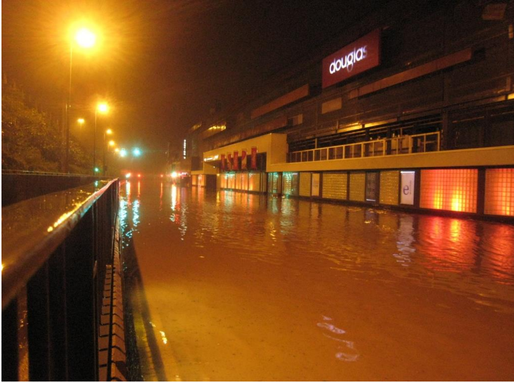
Figure 2.9: Post 2012 flood event outside Douglas Village Shopping Centre. Source: Cork County Council
