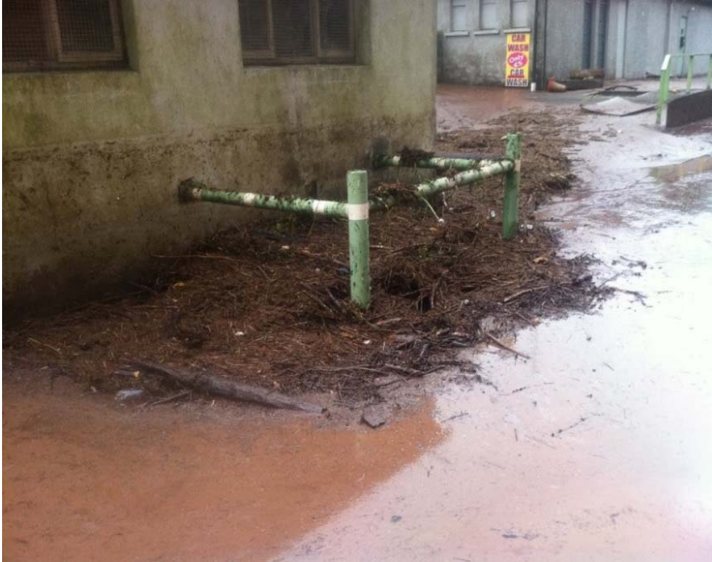
Figure 8.12: Post 2012 flood event adjacent to Donnybrook Commercial Centre showing manhole blockages (Source: Donnybrook Commercial Centre)
