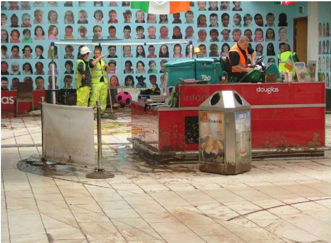
Figure 8.10: Post 2012 flood event inside Douglas Village Shopping Centre. Source: Cork County Council
