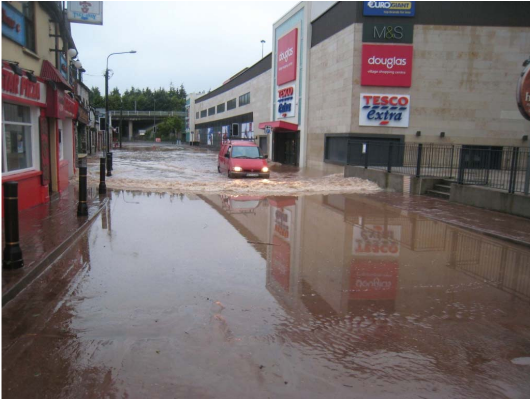
Figure 8.11: Post 2012 flood event in Douglas Village Centre. Source: Cork County Council
