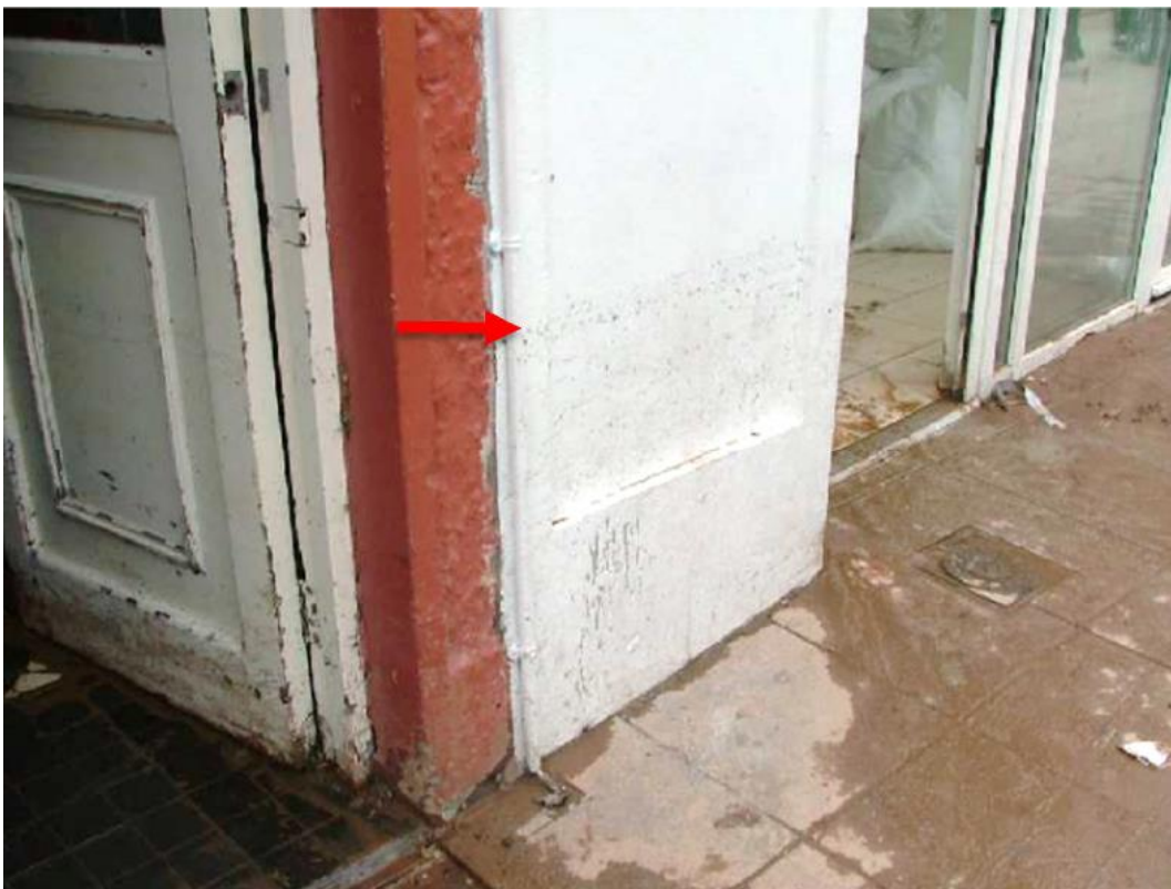
Figure 2.7: Post 2012 flood event high water mark from outside commercial property in Douglas East. Source: OPW
