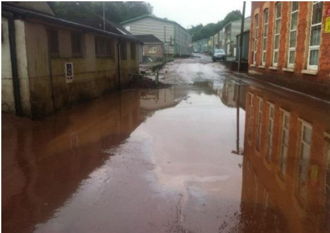
Figure 2.13: Post 2012 flood event at Donnybrook Commercial Centre. Source: Donnybrook Commercial Centre
